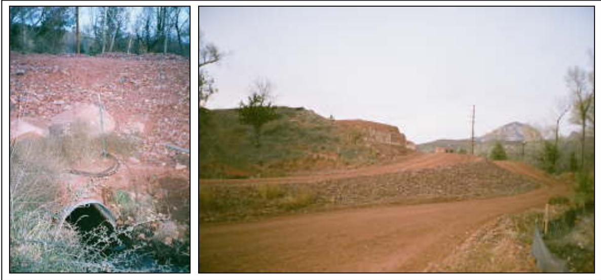
**Photo 2.** Red Rock Ditch showing new culvert and unauthorized fill from road construction. The ditch runs under the new road in right-hand photo
