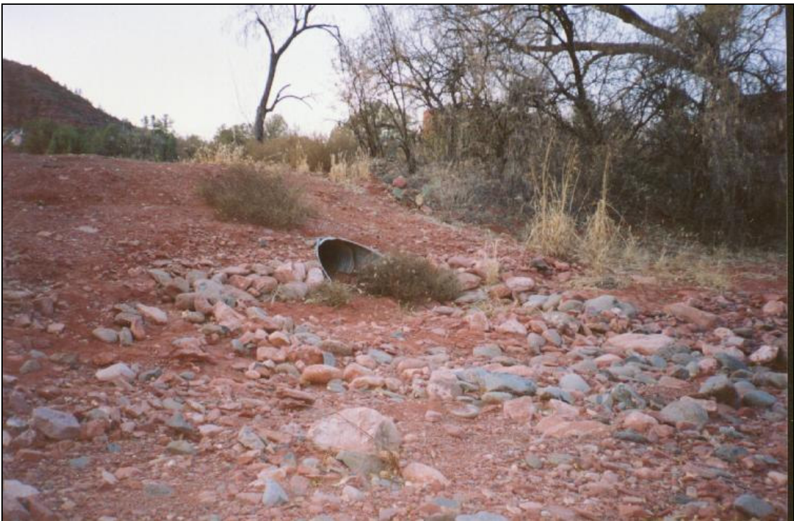
Photo 3. Culvert constructed in jurisdictional area of Carroll Canyon Wash
