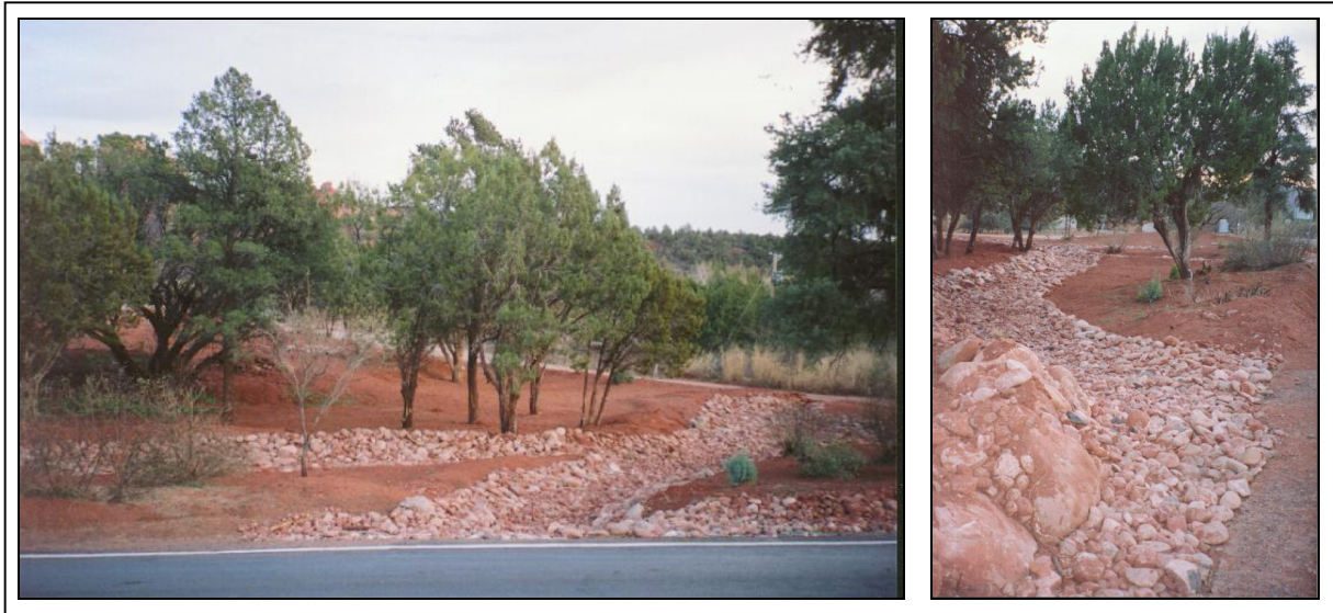
Photo 4. Fill in upland tributary water of the U.S.
